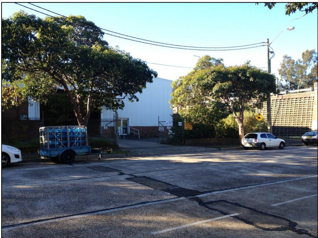
Figure 5: The existing 2-storey warehouse building as viewed from Epsom Road
