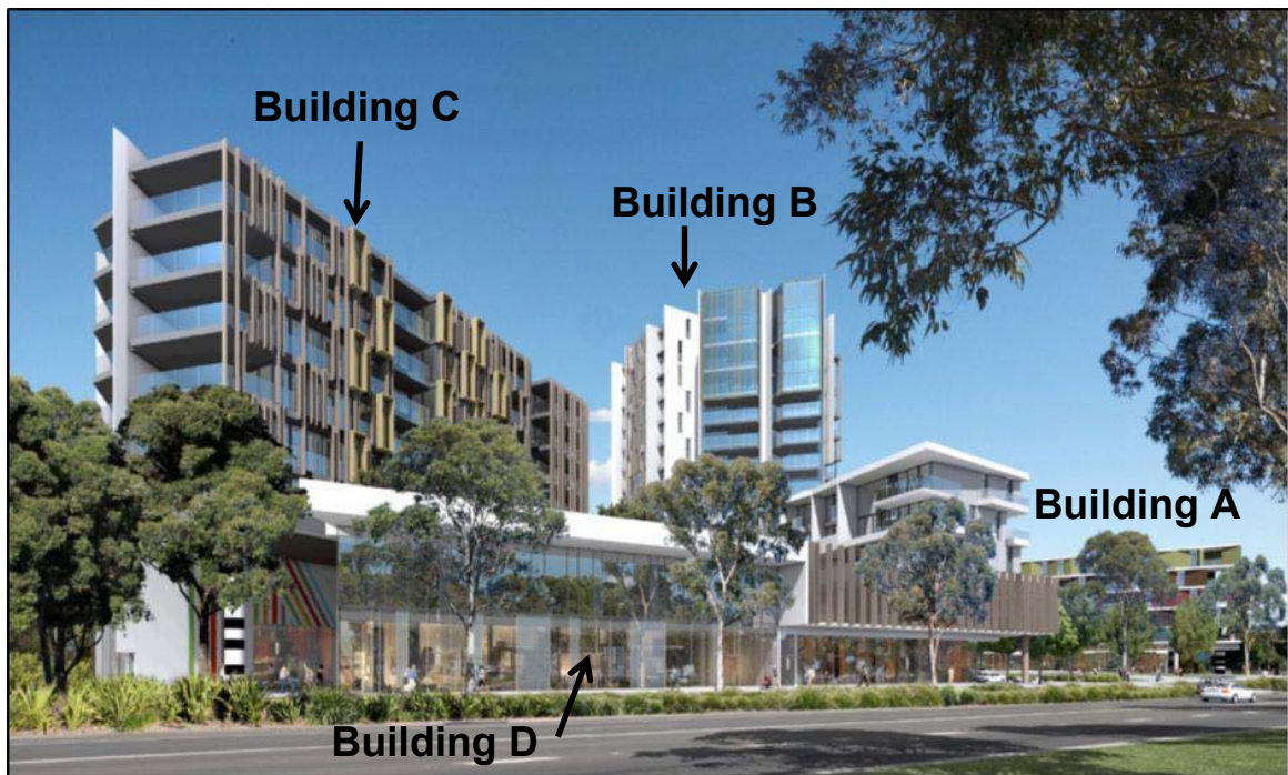
Figure 14: The western elevation of Buildings C and D and northern elevation of Building B as viewed from Link Road
